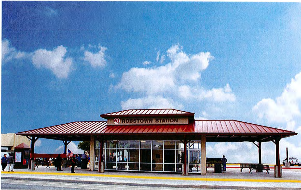
Robstown Transfer Station
